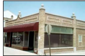
Commercial Building – Built 1926 - 125 S. Villa Ave.
